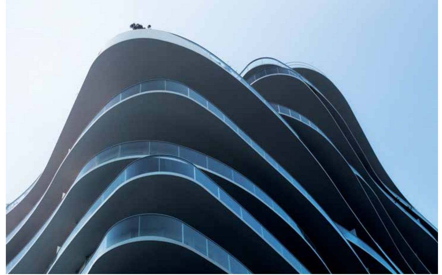
UNIC Residential emerges as part of the mixed-use masterplan envisioned adjacent to the Martin Luther King Park – a 10-hectare green space. © Arch-Exist.
